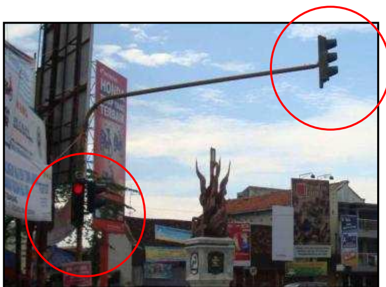
Poor Condition of Traffic Signals (Damaged and Broken) and Pedestrian Crossing Blocked by the Poles
