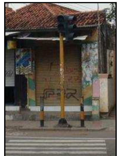
Poor Condition of Traffic Signals (Damaged and Broken) and Pedestrian Crossing Blocked by the Poles
