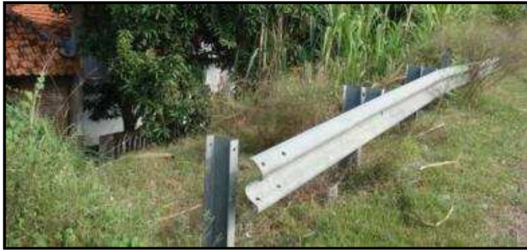
Broken Guardrail and No Maintenance
