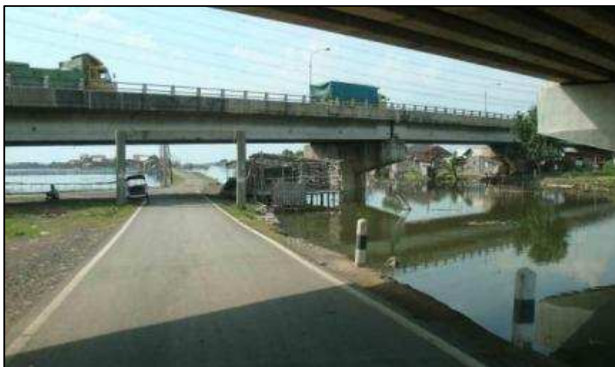
Poor Signing & Inadequate Delineation or Protection at Water & Below
