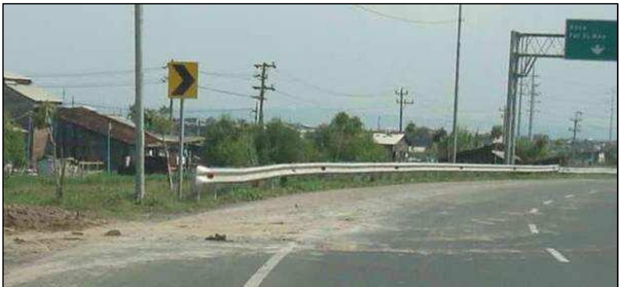
Exposed but Protected end of Guardrail at start of bend
