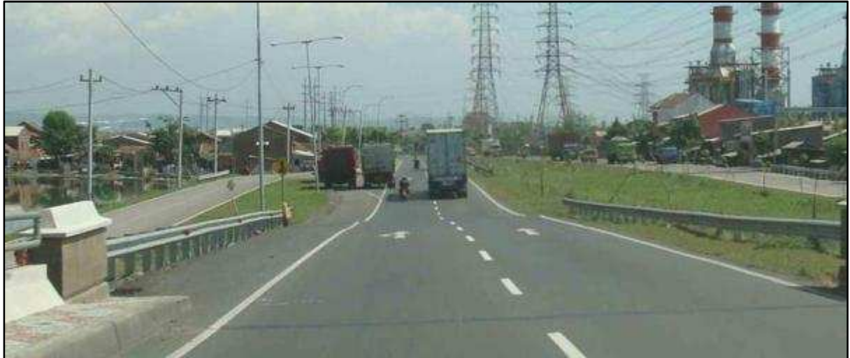
Exit to Local Road Unsigned & Hidden by Parked Trucks
