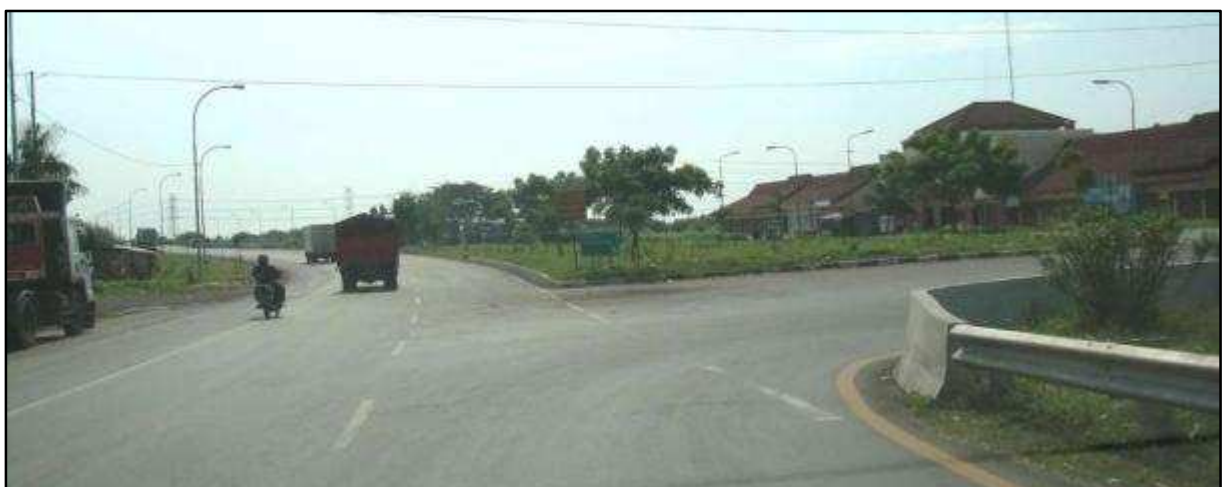
Unclear Signing & Markings at U Turn - Close Up Below
