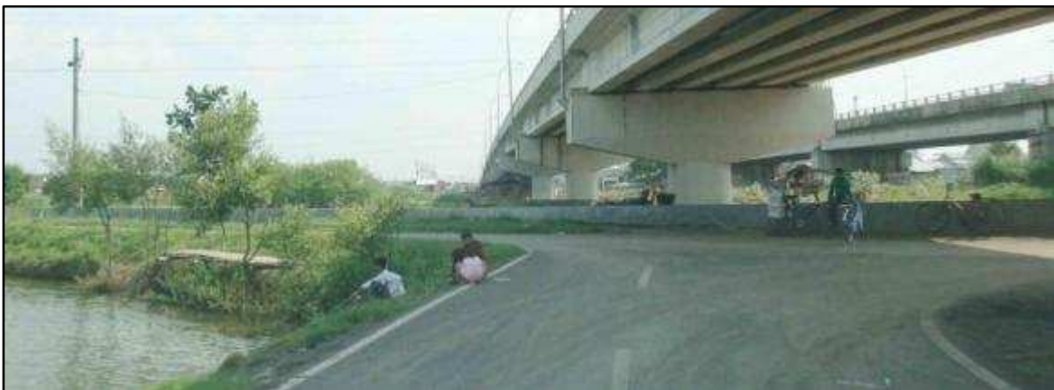
Local Road - Lack of Delineation & Signs
