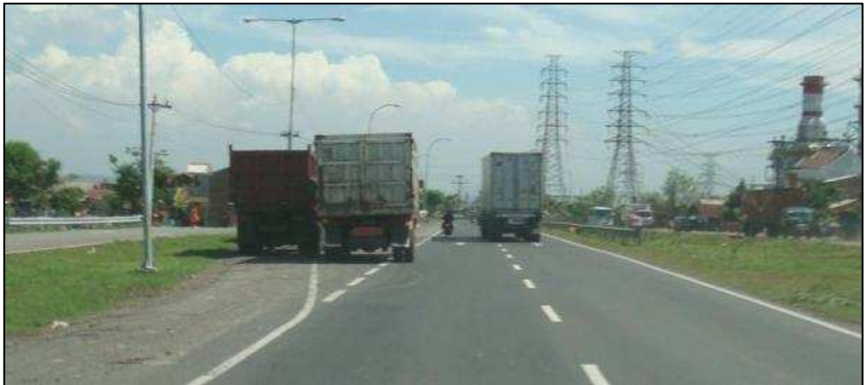
Exit to Local Road Still Hidden & Blocked
