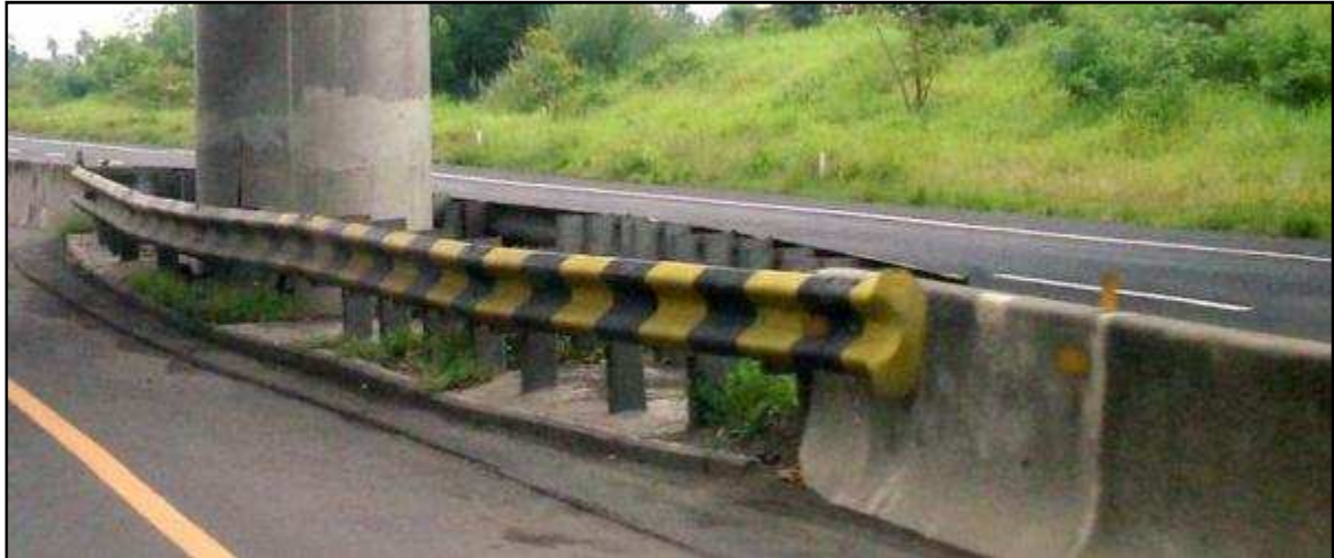
Overlap Between Guardrail & Concrete Median on Indonesia Tollway
