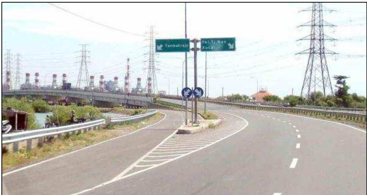
High Standard Signing of Exit to Local Road
