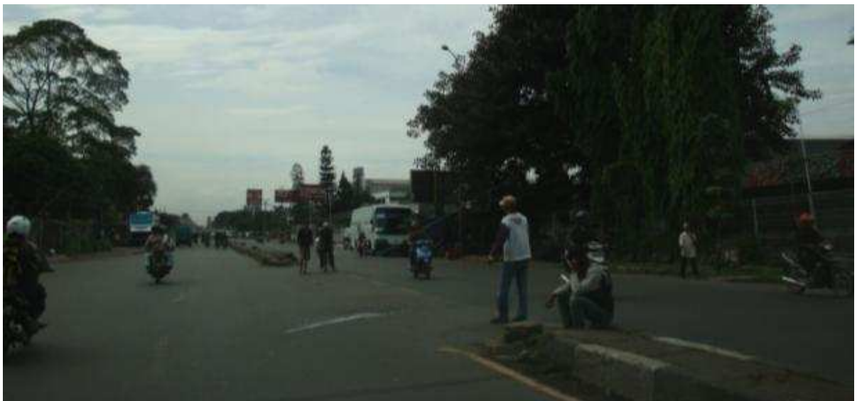
Gaps on the narrow median (difficulties to make U turn)
