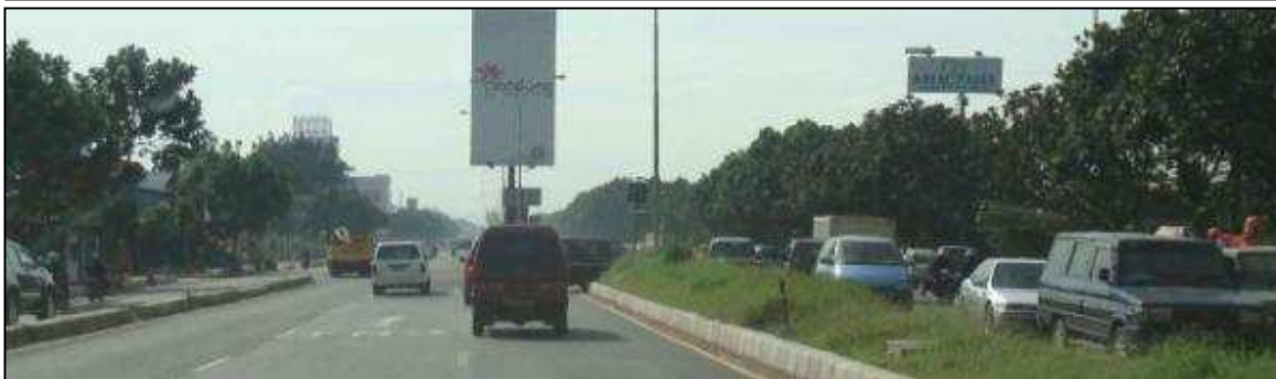
No taper for making the U turn, the vehicles could be crashed from behind
