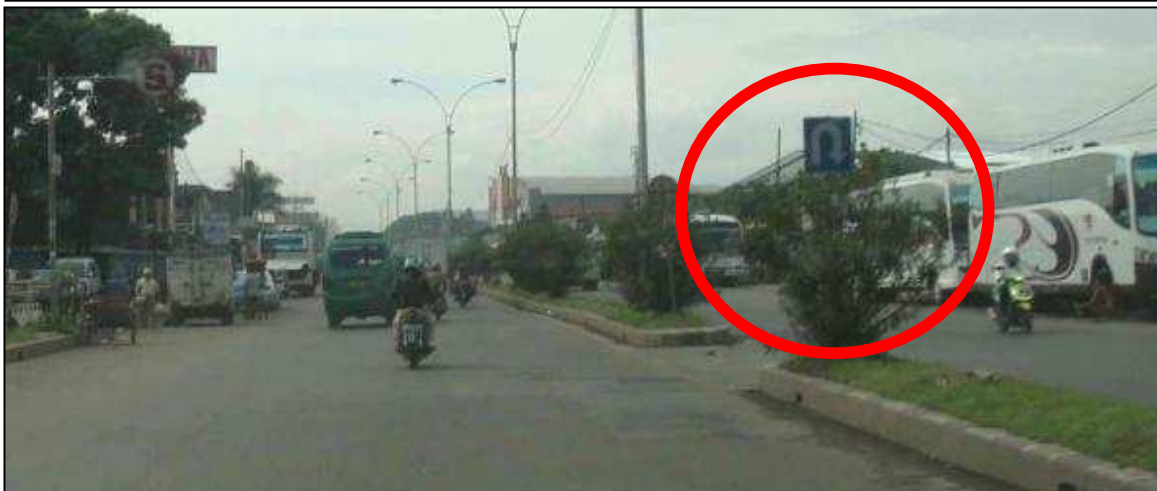
Median is too narrow, bus parked on the main road, the road sign will be cover by plant in a short time, the visibility of vehicles which Turning was blocked by trees
