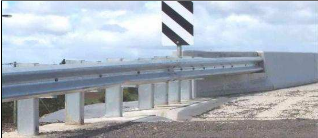
A proper connection between guard rail and parapet
