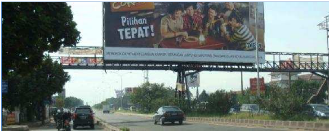
The pedestrian bridge was not protected by guard rail
