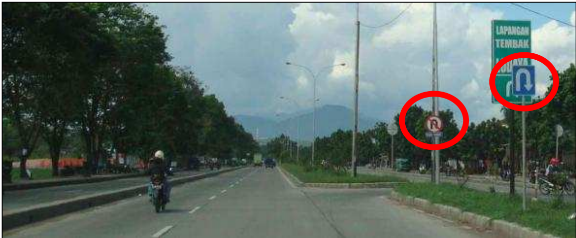
Two different sign for U Turn makes the road users confused, and U Turn service already have taper
